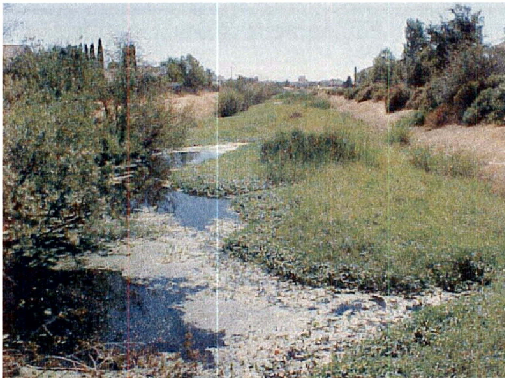
Photograph 2 Strawberry Creek is a channelized perennial stream in northern Elk Grove that is nearly choked with fresh emergent wetland vegetation. This photograph is taken from Sheldon North Drive, looking north.
